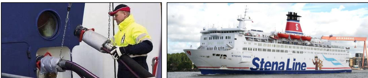
Figure 9-14: Connection of the district heating solution on the docked “Stena Danica” in order to replace the use of diesel in oil-fired boilers (Norsk Fjernvarme, 2018).
